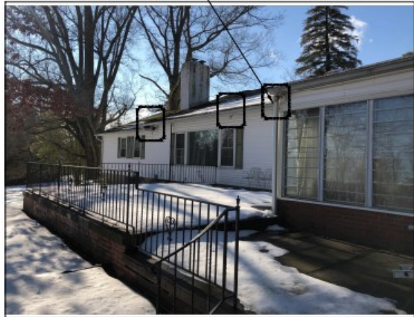
③ EXISTING REAR OF BUILDING N.T.S.
